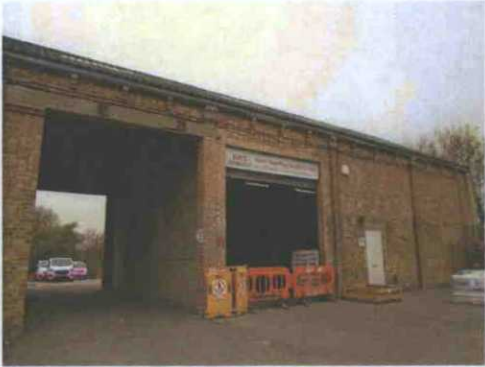
Building B2b, from the east
