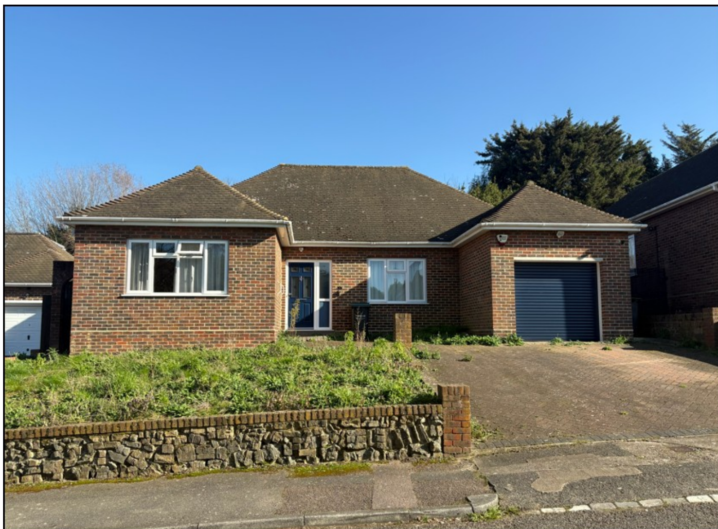
Site Photo taken on 18.03.26
