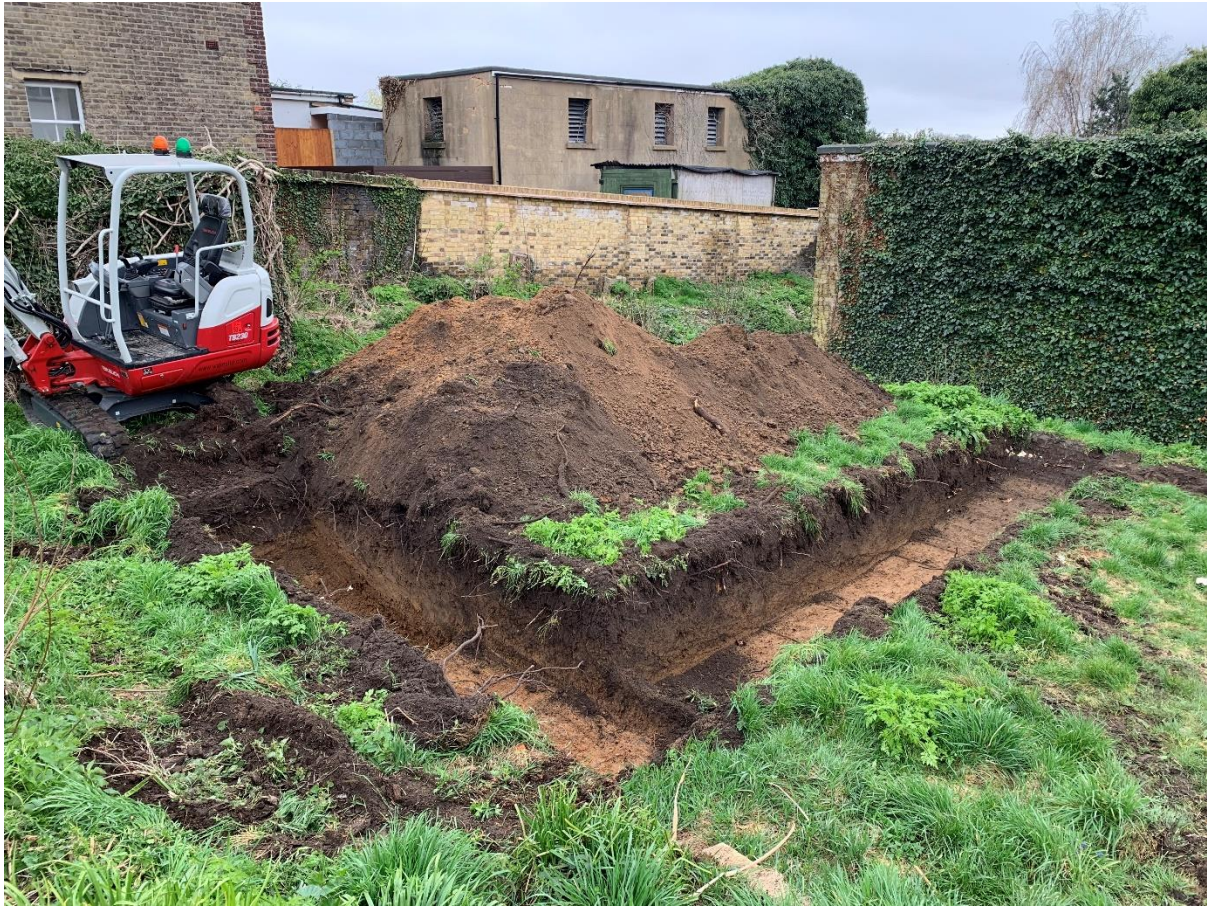
Figure 9: General view of Trench 2 looking south-east, with the hall to the right.
