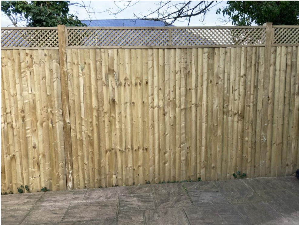
EXISTING FENCE PANEL
