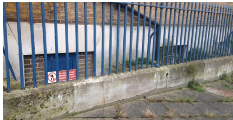
Photo of side elevation light wells
