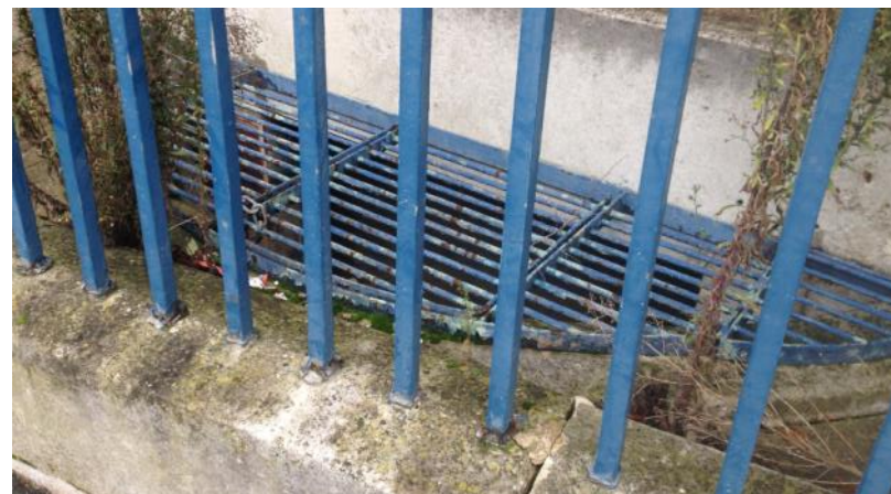
Photo of front elevation light well
