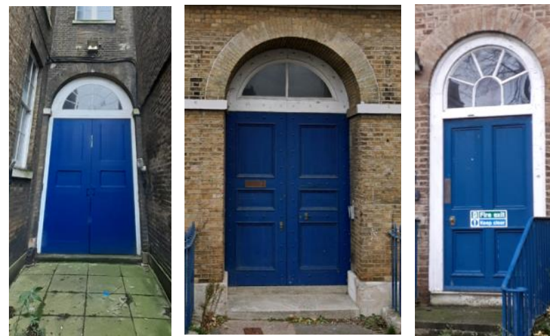
External doors to be refurbished and retained.
