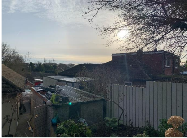
Rear No 50 garage Looking towards No 48
