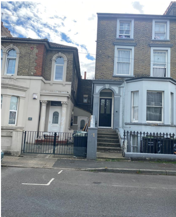
Single & Two Storey Side Extension – 16 Darnley Street
