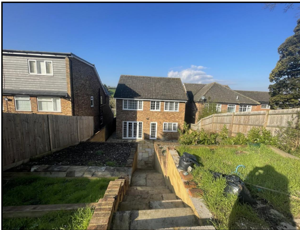
Image of Rear Elevation taken during the site visit
