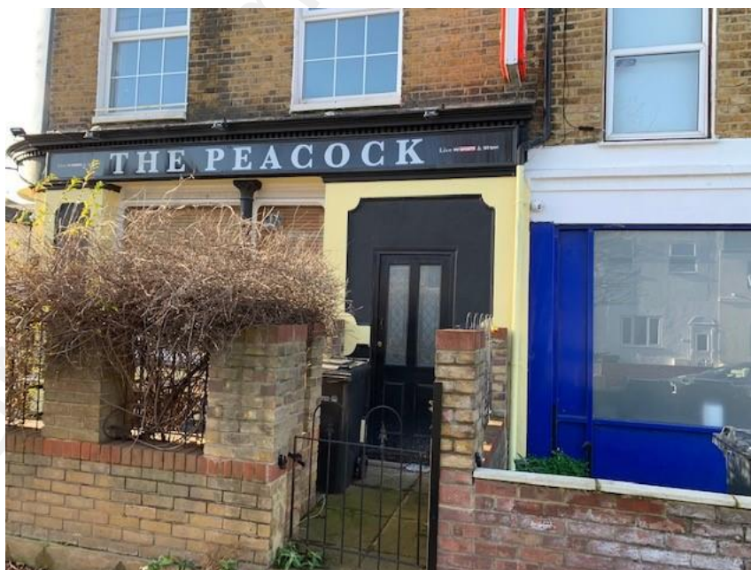
P04 – View of residential entrance and residential refuse area of 78 Peacock Street
