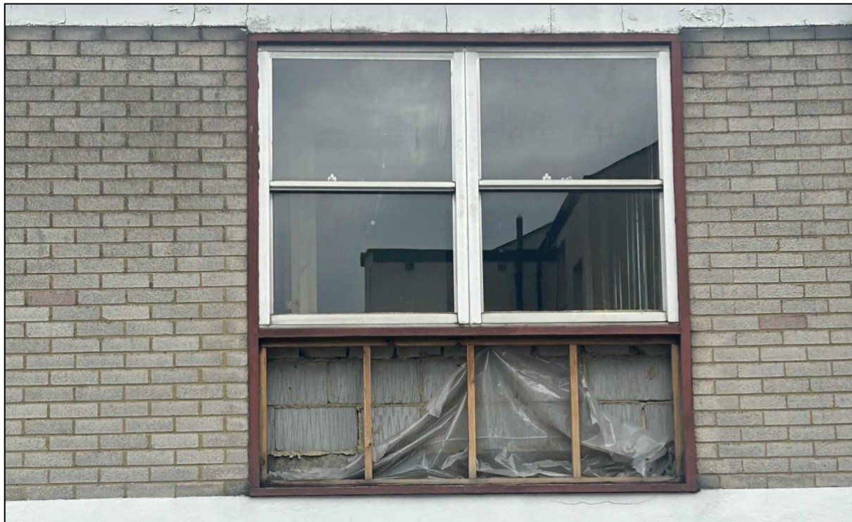
Figure 4 – Existing window with wooden panelling partially removed.
