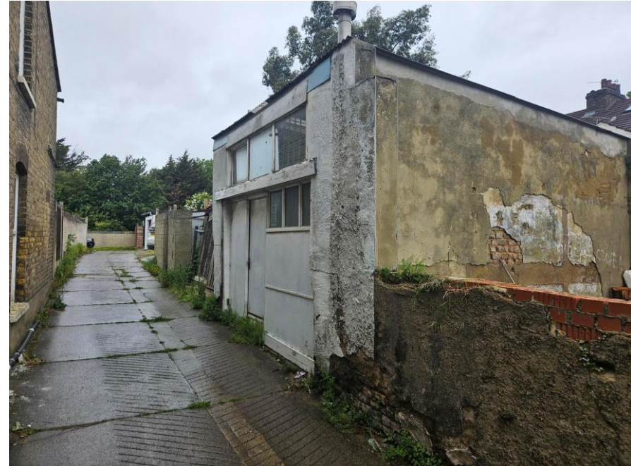
Figure 1: View of the existing rear workshop
