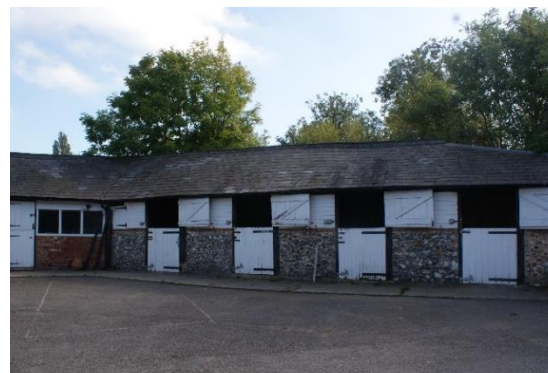
Figure 2.5: Disused stable building
