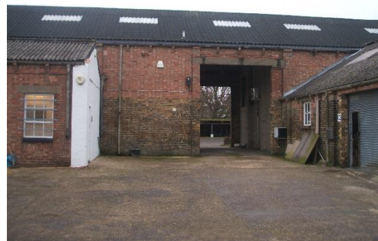
Figure 2.3: Existing industrial buildings
