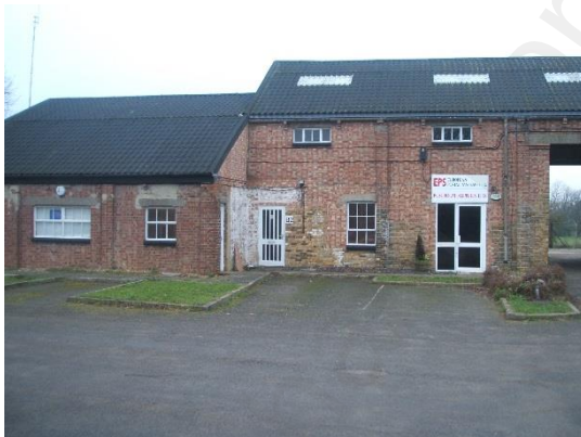
Figure 2.2: Existing industrial buildings
