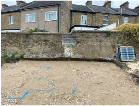
PLAQUE LOCATION AS SEEN APPROACHING FROM ARMOURY DRIVE
