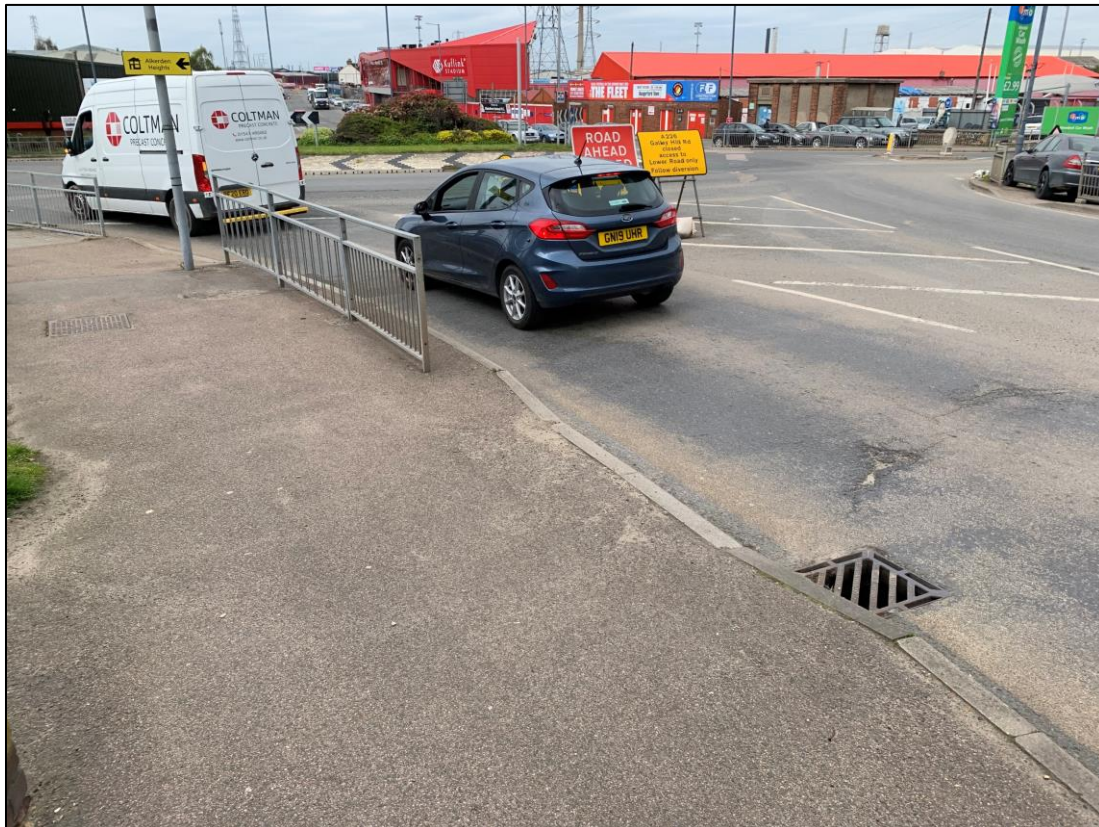
Photo 7: Dropped kerb crossing point (B2175)
