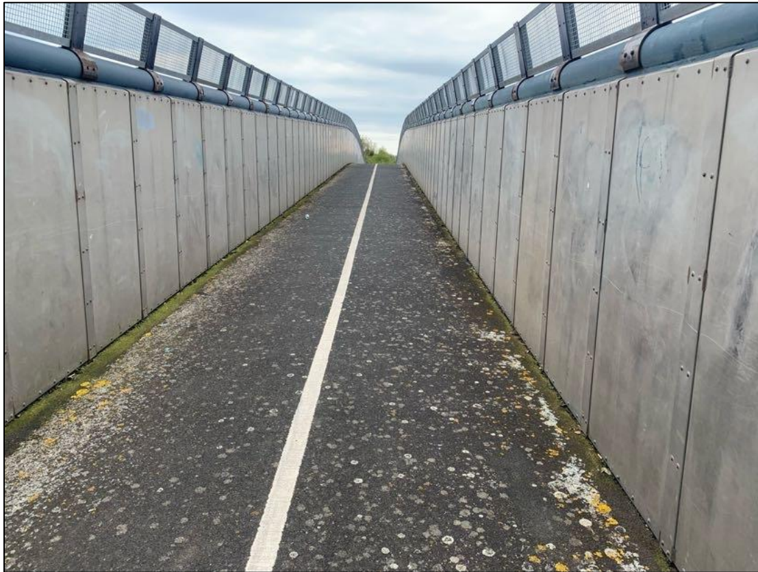
Photo 13: Shared path over railway tracks
