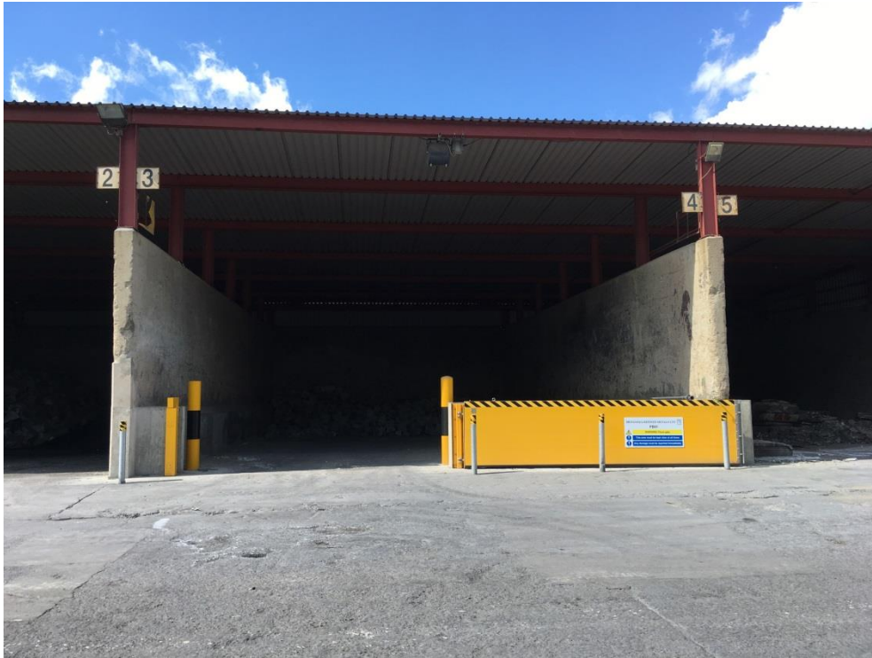
Example of a Flood gate
