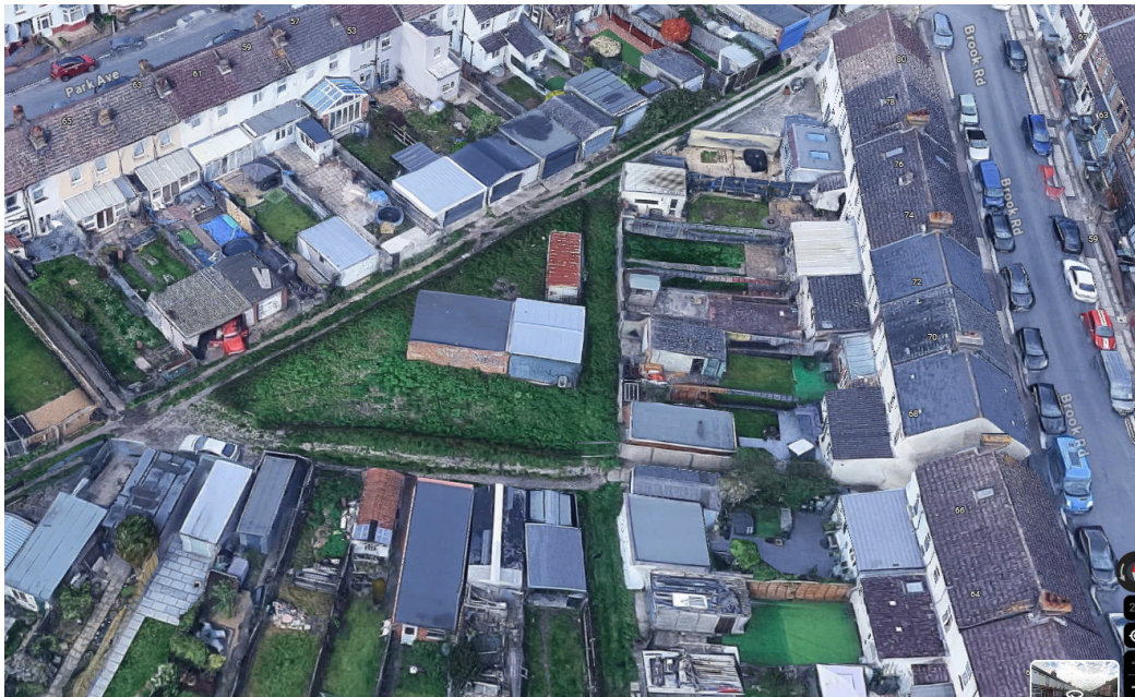
P004 – aerial view of existing site looking north
