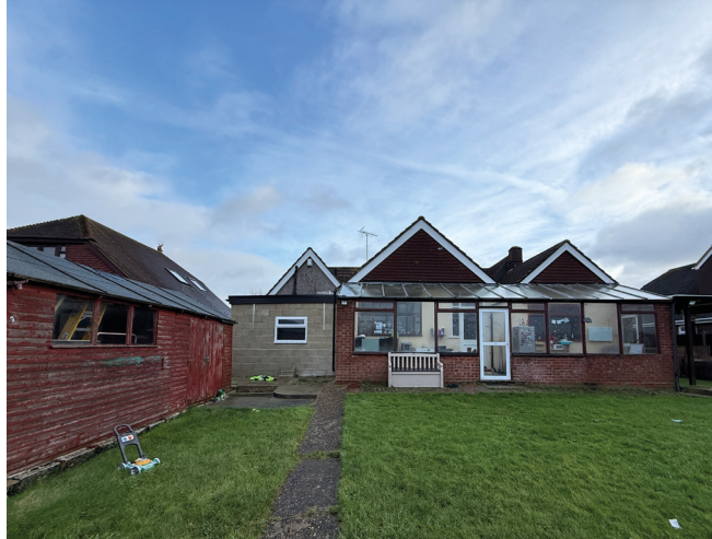
Fig.4 - Rear elevation of site showing existing extension
