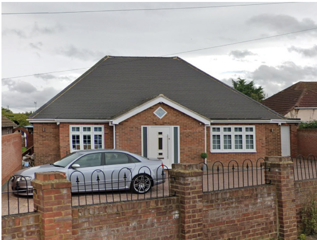
Fig.11 - Brick bungalow with central gable-end and slate tiles
