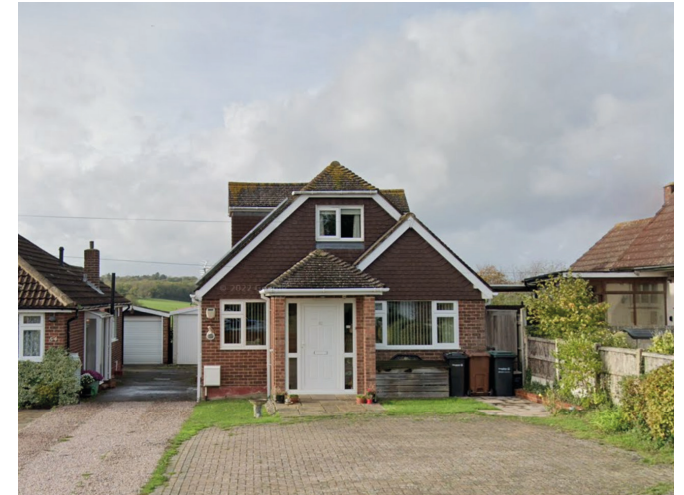
Fig.10 - Neighbouring property (No. 52) with red brick and tile
