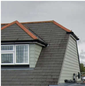
Slate Roof on Lewis Road
