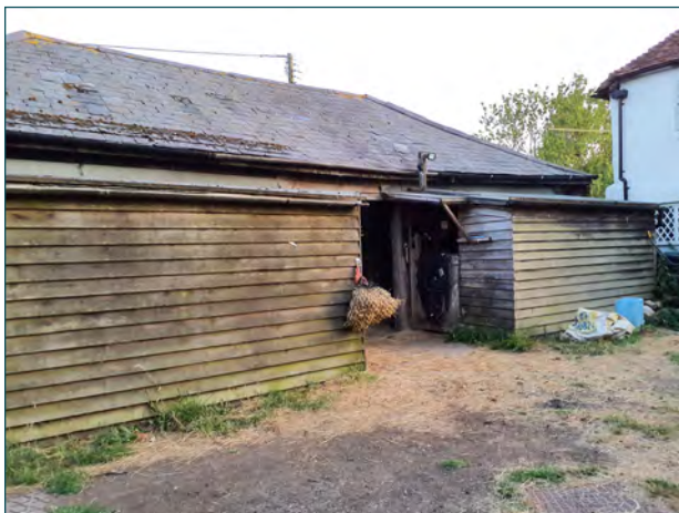
Photograph 1. Northern elevation of Building B1
