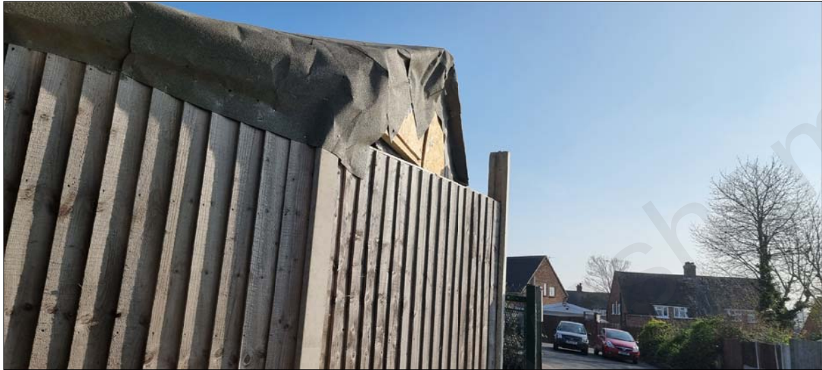
North Side boundary (rear)
