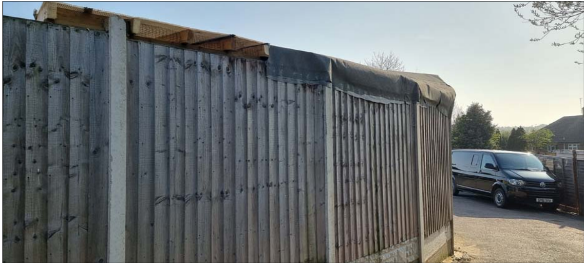
North Side boundary
