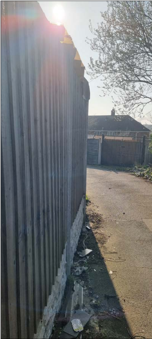
North Side boundary
