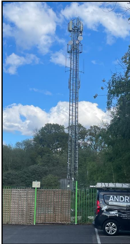
Taken on site on 29 th March
