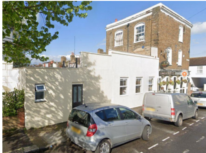
Existing Side View
