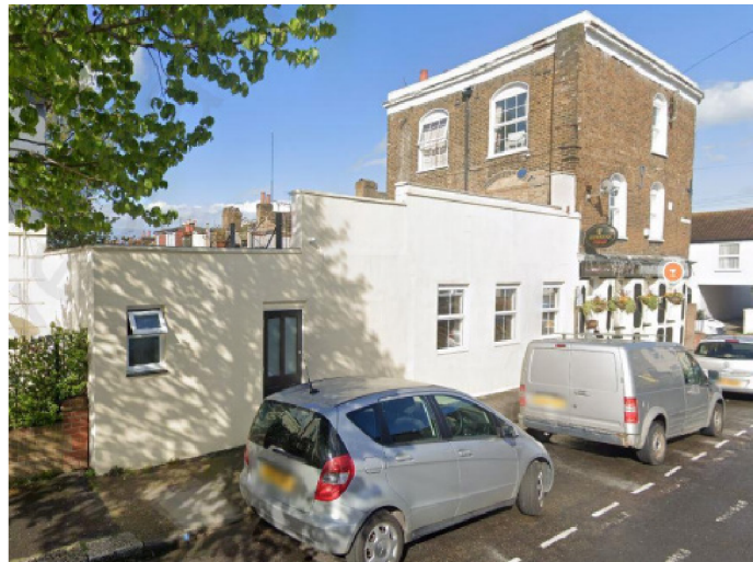
Existing Side View
