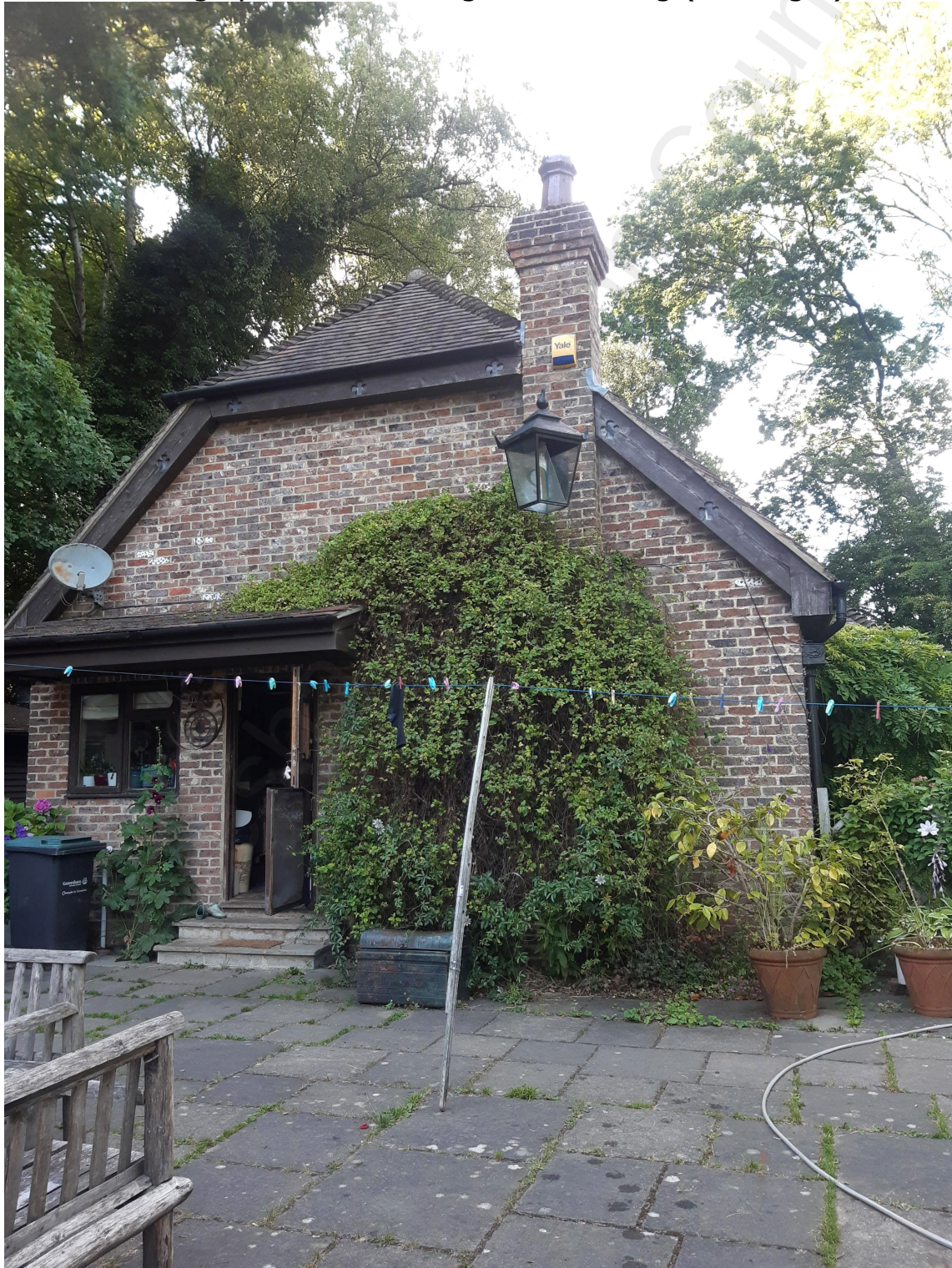
Photograph of the existing Host dwelling (7m height)
