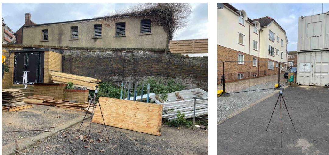
Figure 3: Picture of the Measurement Positions (MP2 - left) and (MP3 – right)
