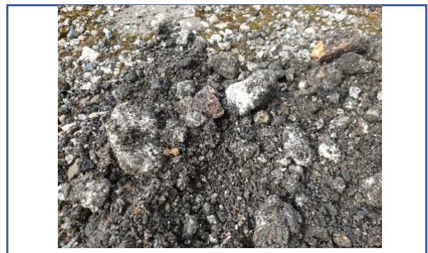
BH201 arising to 2.7m bgl
