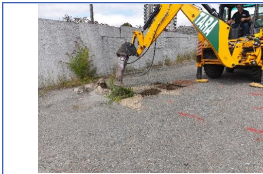
Manhole cover west of the subject site
