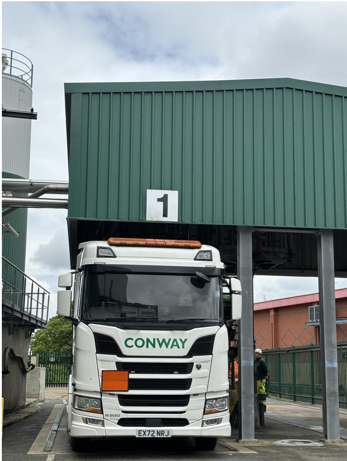
Figure F7 Lorry Loading within the Existing Loading Gantry (3)
