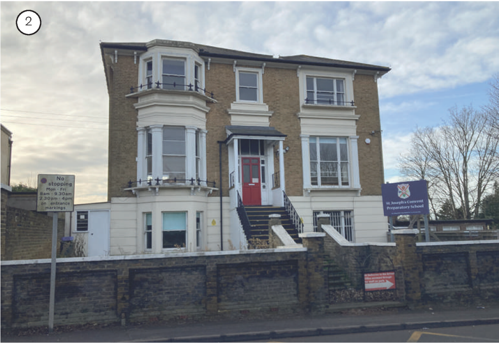
Building to be retained
