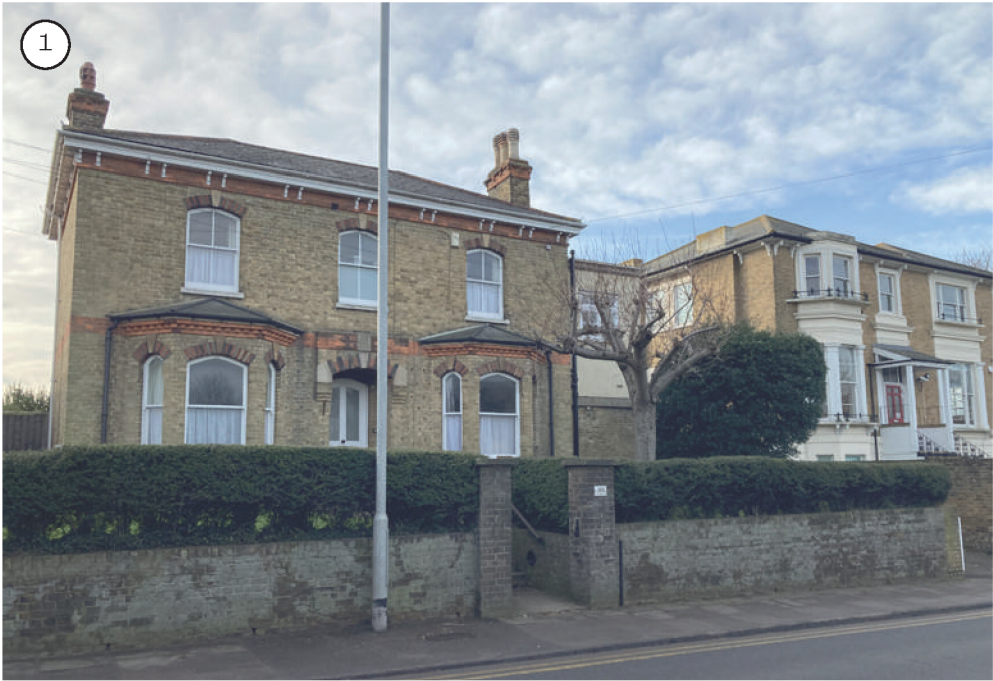
Front facade of St. Joseph's Covent Preparatory School
