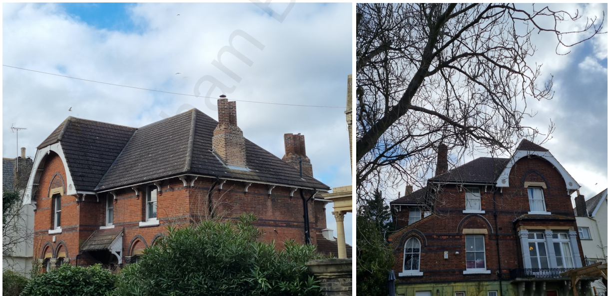
Figures 1 & 2. Views of the front and rear of the property.
