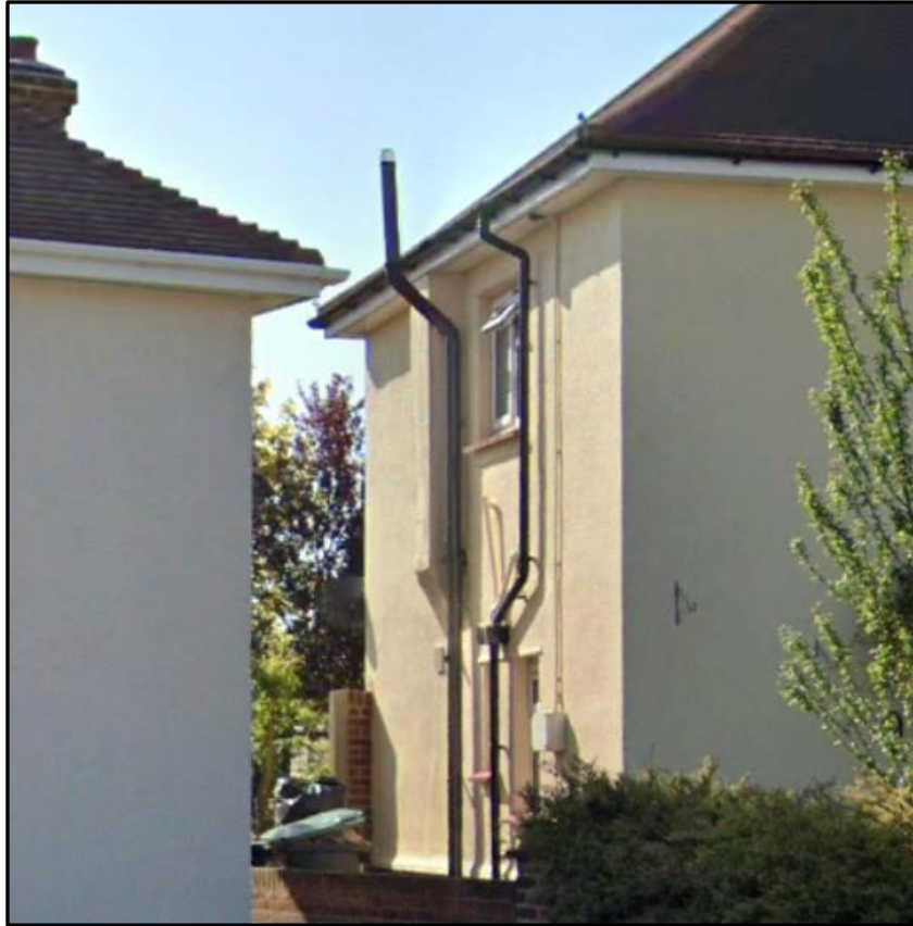
Neighbours side openings.
