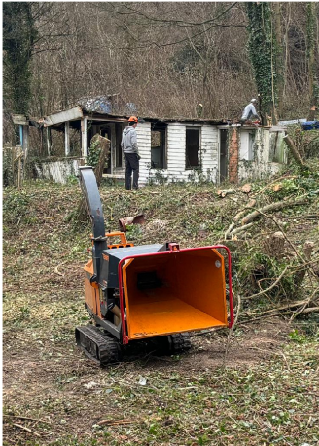
A picture showing the full extent of the existing building before unsafe parts were removed.
