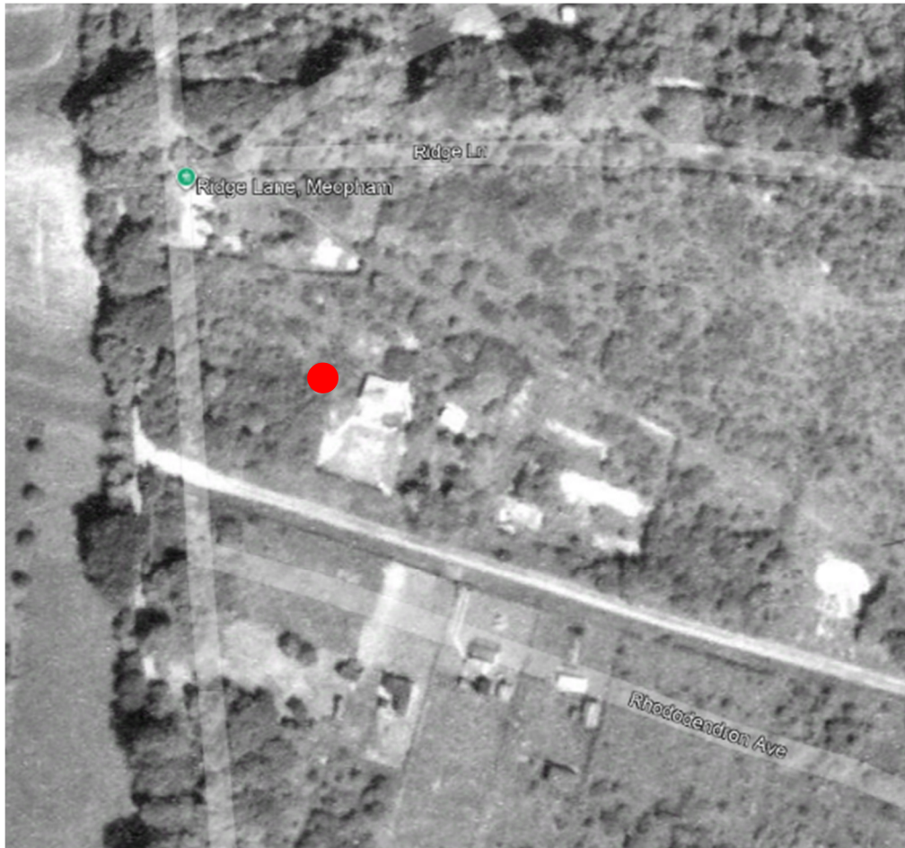
1960 aerial view of the plot and the existing structure in situ.
