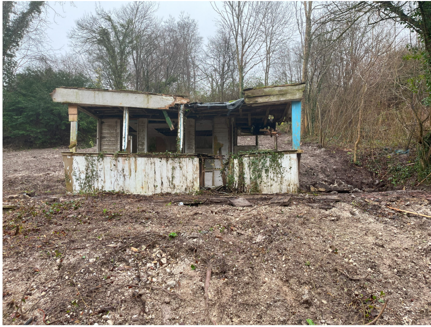
Existing building currently on site.
