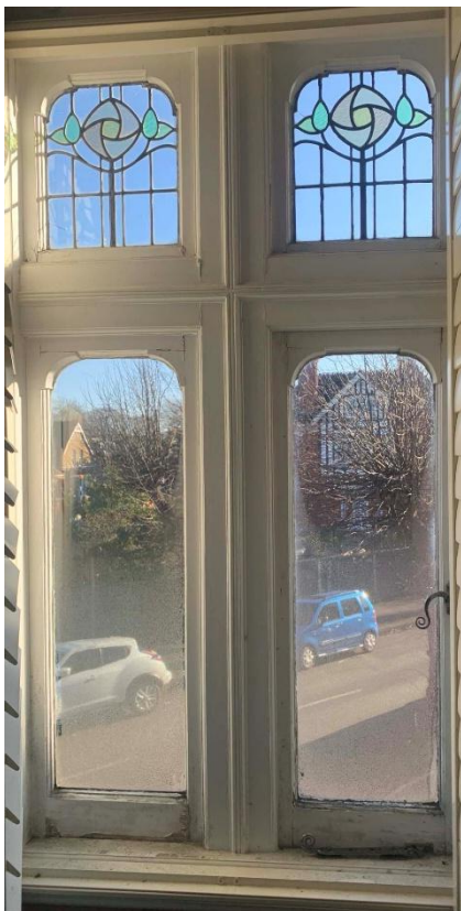
Figure 3: Internal view of one of the first floor turret windows.
