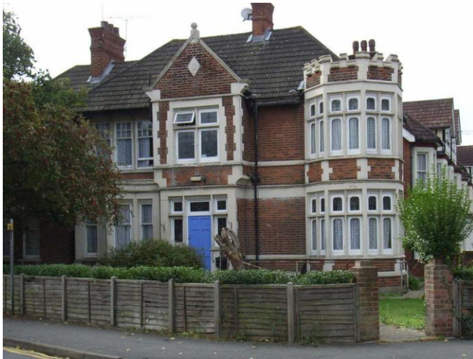
Figure 1: 1 The Avenue, October 2011
