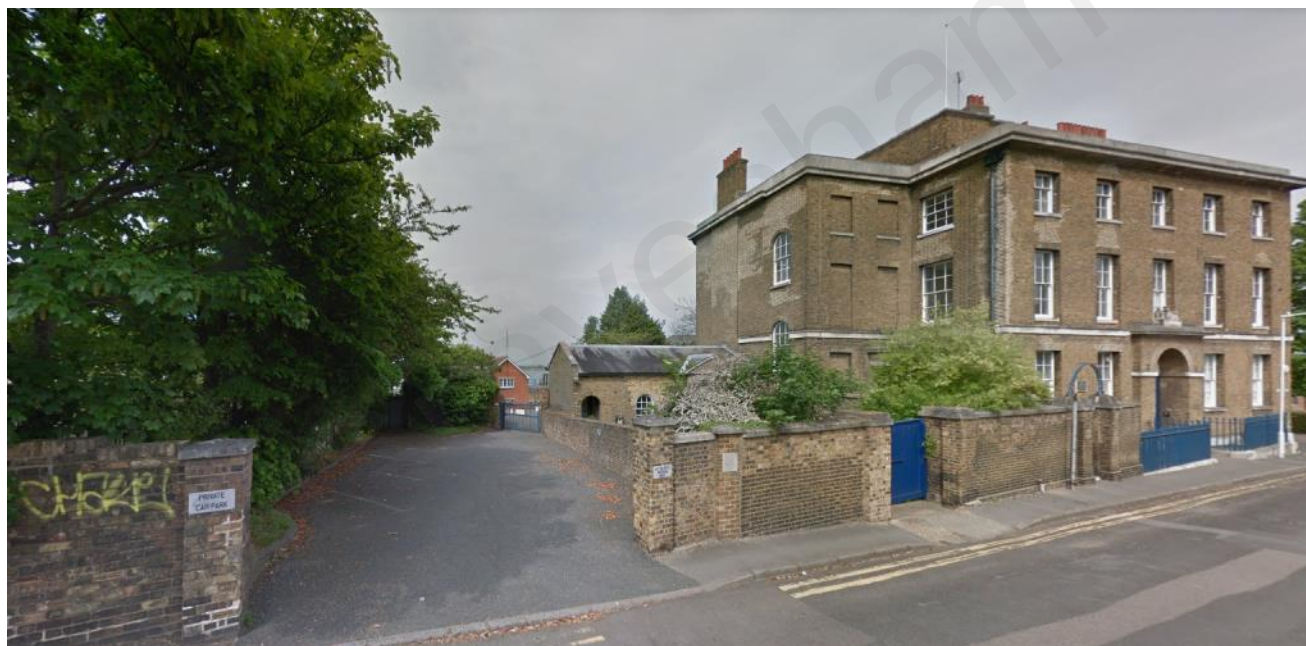
View along the sites southern boundary, with the front elevation of Custom House and the access from The Terrace visible.
