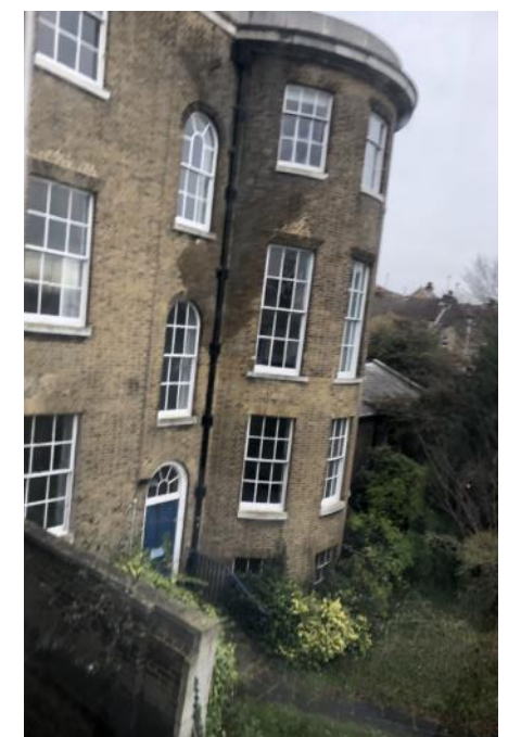
Rear of Custom House
