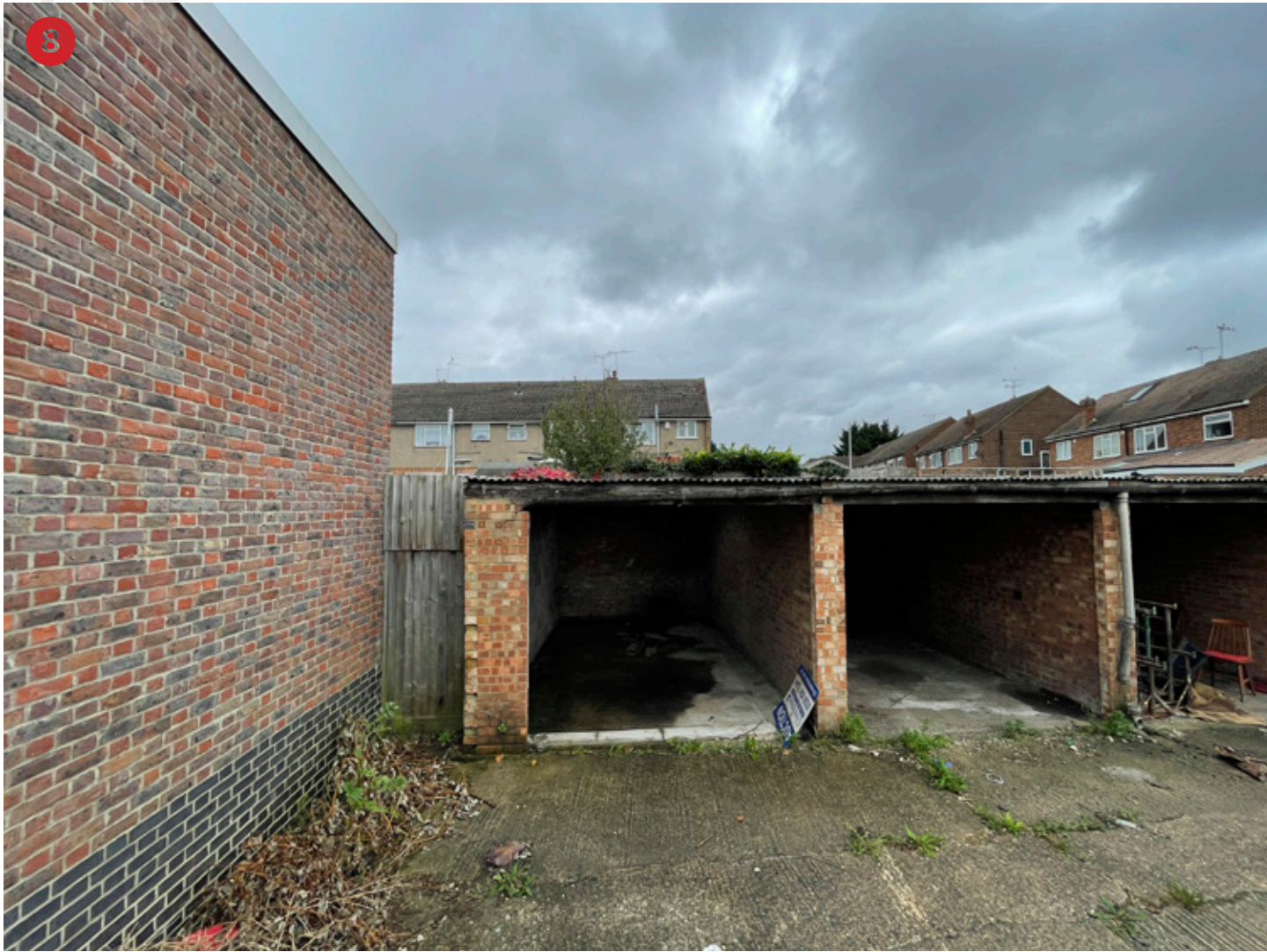
View looking towards the houses on Pirrip Close
