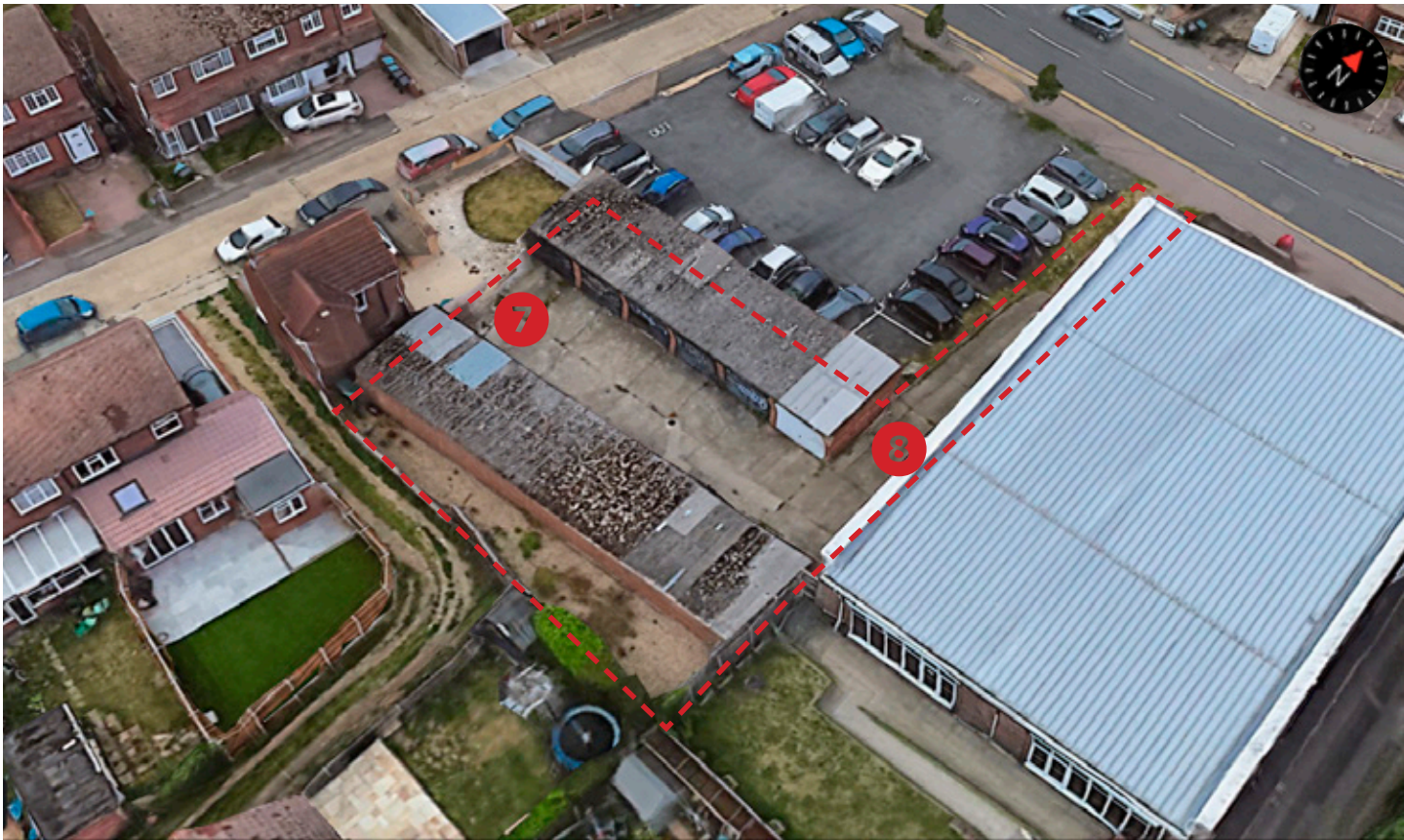
Aerial view of the site
