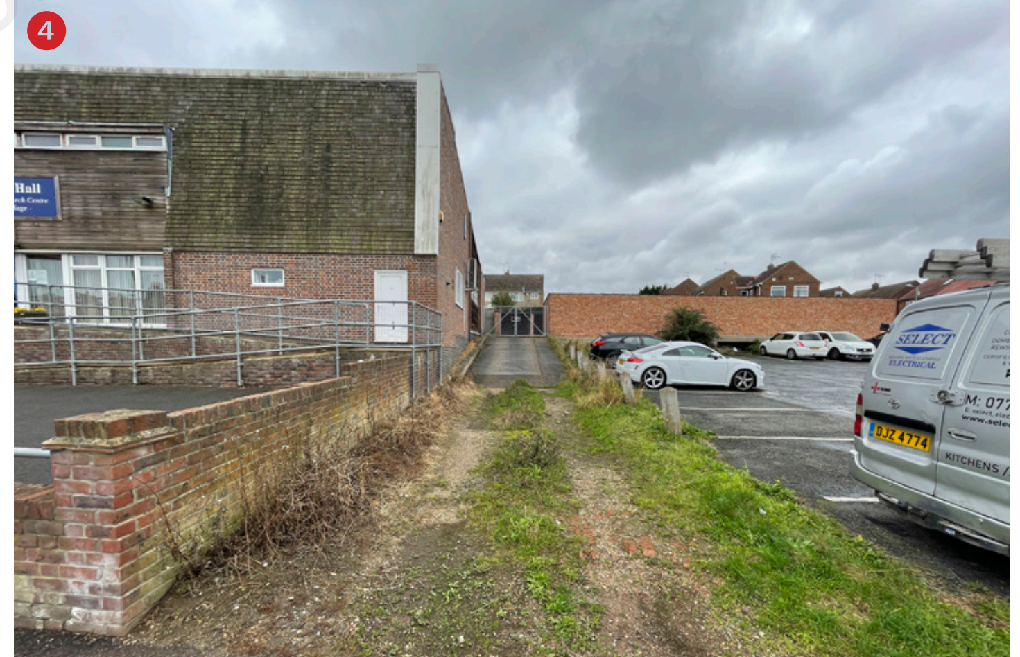
View from Lower Higham Road, viewing the driveway to the garages
