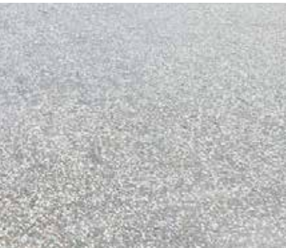
In situ exposed grey aggregate poured concrete
