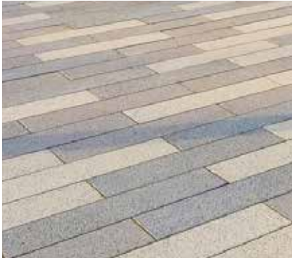
Buff tone rectangular concrete flags
