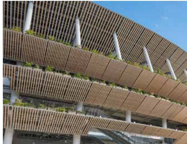
Japan National Stadium - Kengo Kuma
