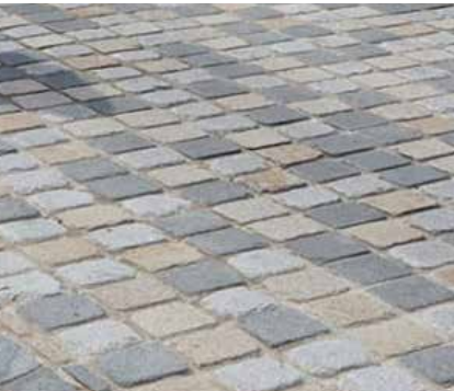
Tumbled vehicular sett paving, buff tones
