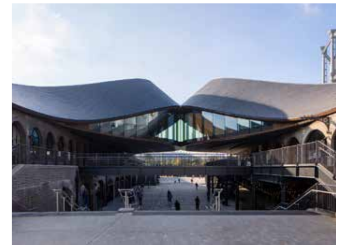
Coal Drops Yard - Heatherwick Studio
