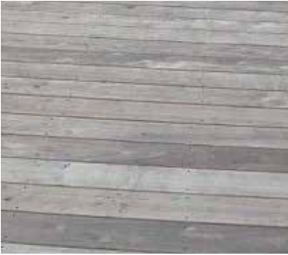
Composite timber decking
