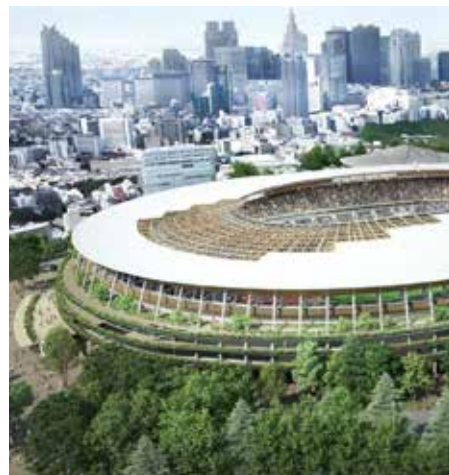
Japan National Stadium - Kengo Kuma
