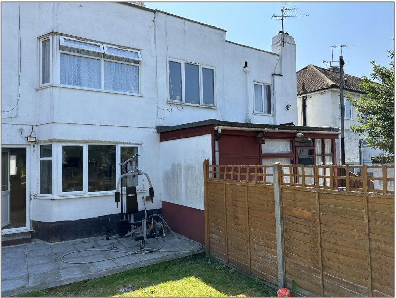
Rear view to neighbour rear extension
