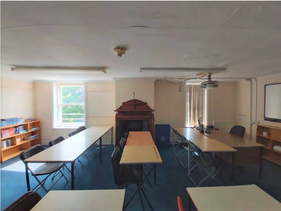
Ceiling of HSFX06 H1 classroom looking east Photograph taken 01/08/2022 by CP
