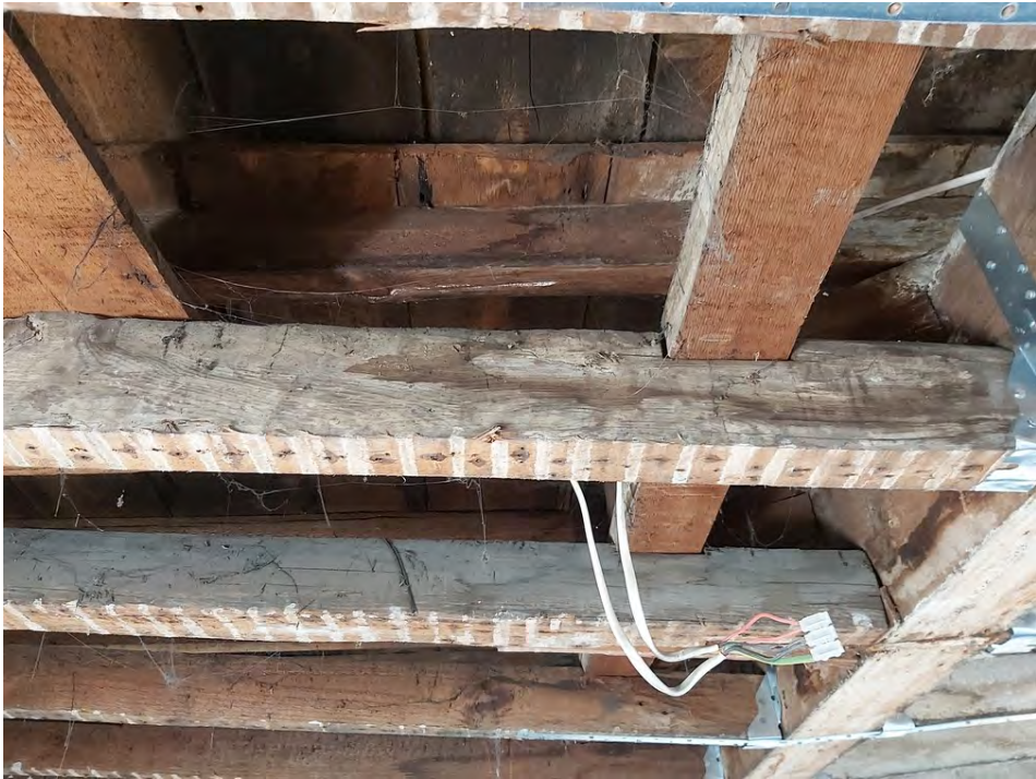
Ceiling of HSF06 H1 classroom looking north Underside of lead roof RFX03. Photograph taken 23/11/2022 by CP
