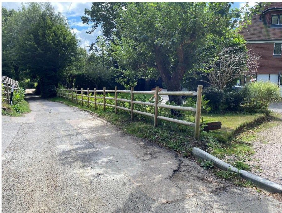
FENCE AND HEDGE ADJACENT TO BOWESDEN LANE
