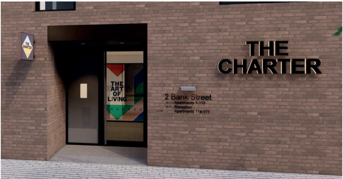
Block E01 North Façade/Bank Street (West)
