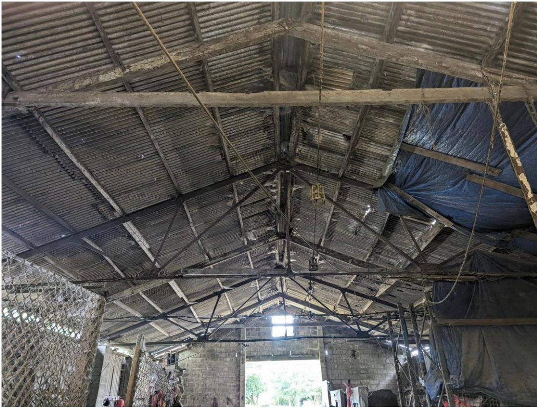
General Internal Photos of the Main Building.
