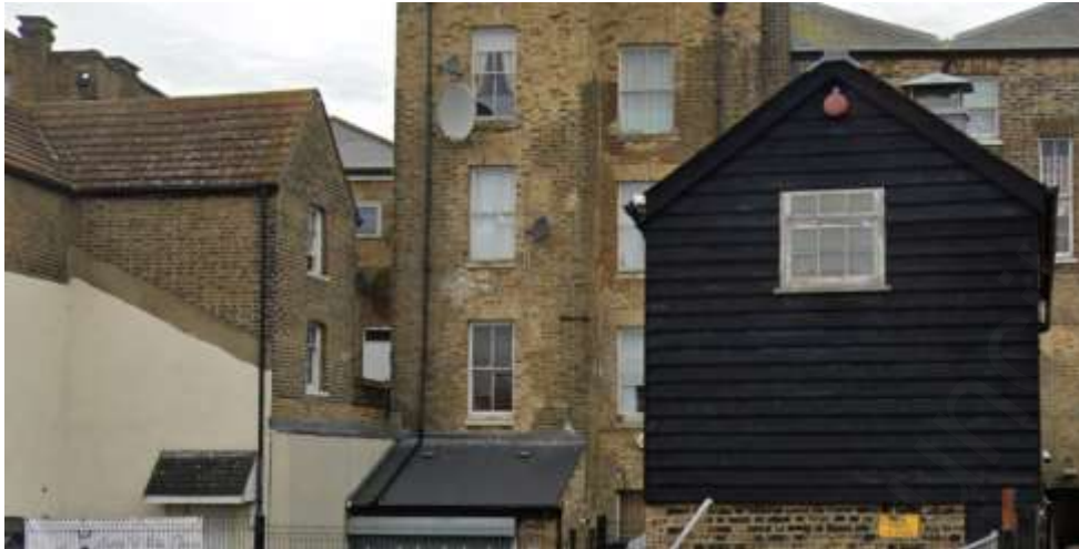
TIMBER CLAD ADJACENT BUILDING
