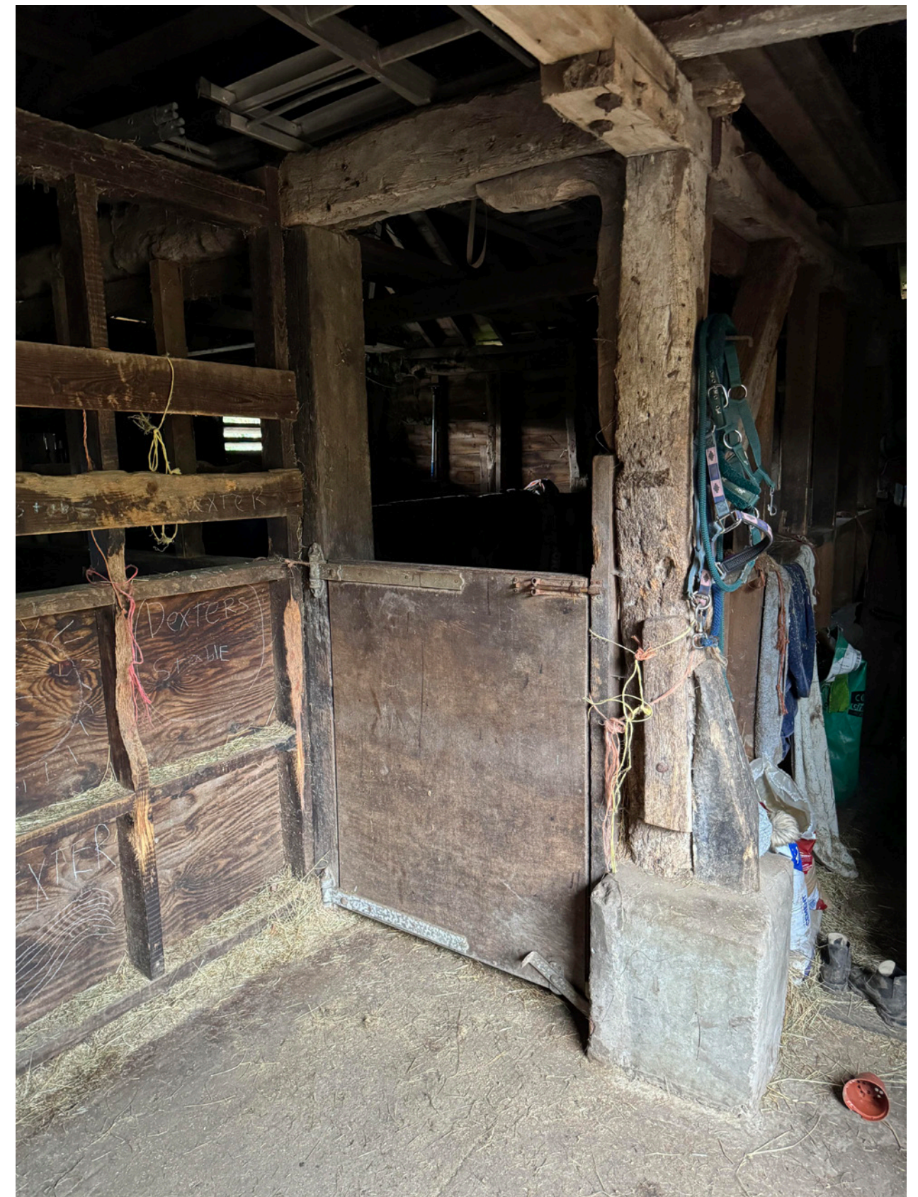
Fig 8 | View of historic post and internal structure
