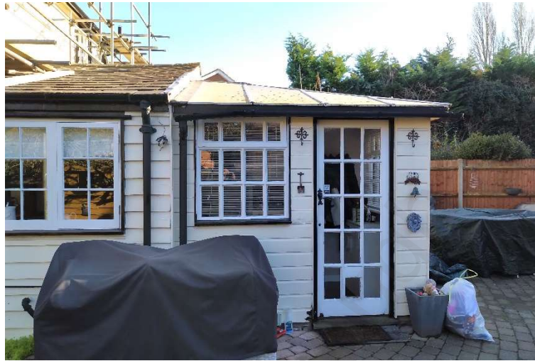
Fig 7. View of the side elevation (conservatory) with Window reference W1 & Door reference D1
