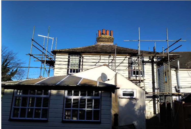
Fig 10. View of the rear elevation (conservatory) with Windows reference W2 & W3
