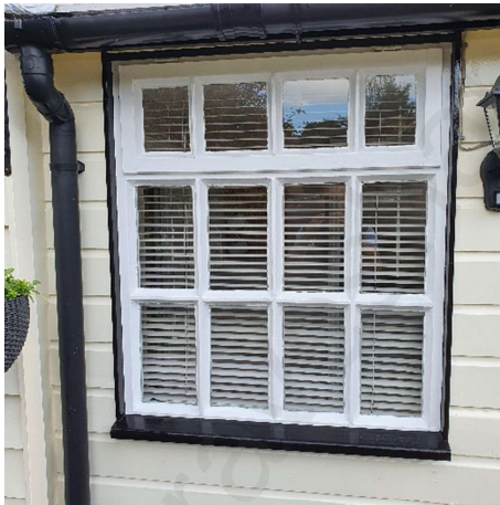
Fig 8. Closeup view of window W1
