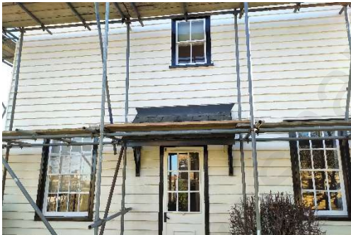
Fig 1. View of the main house at the side
