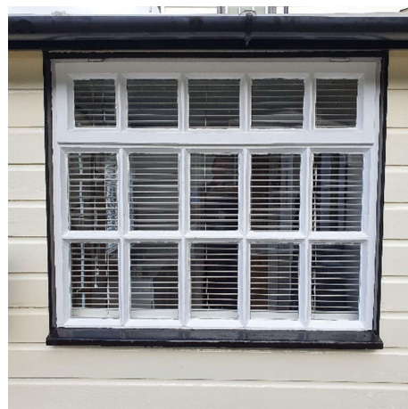
Fig 12. Closeup view of window W3
