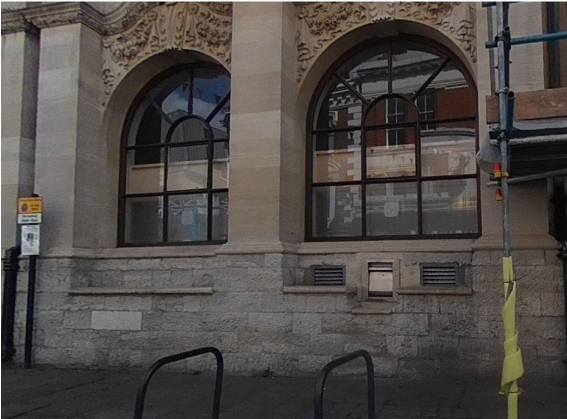
FIGURE 2: EXISTING GLAZED PANELS TO WINDMILL STREET IMAGE:
