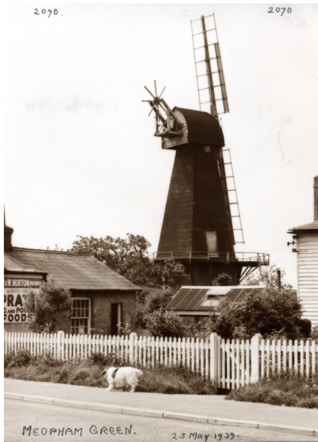
Meopham Mill in 1939, a few years after it ceased working by wind power. Only two sweeps are left and the fantail is a skeleton following storm damage in 1935. (The Mills Archive Harry Meyer Collection)
