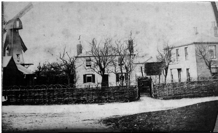
An early photo of the mill, taken during the Killick family's ownership. The fantail has not yet been fitted, and one pair of sweeps is canvas-covered. (Rob Cumming Collection)
