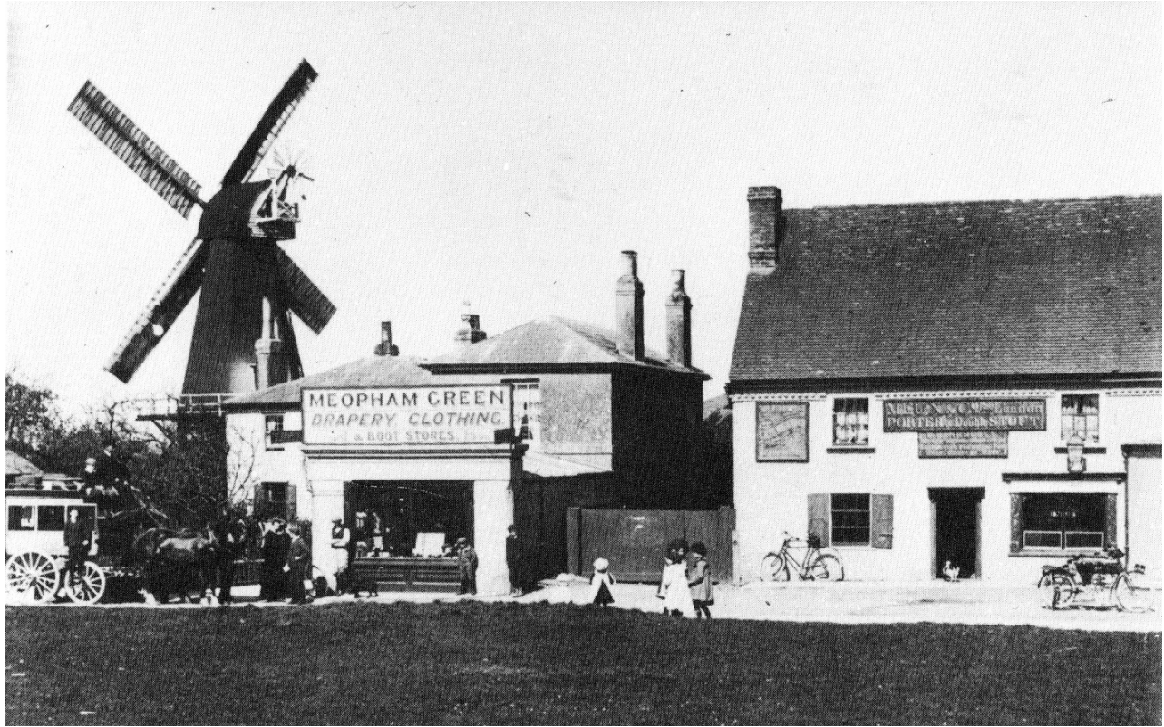
Meopham Mill, c1905, at work with one pair of common sweeps and one pair of shuttered sweeps. A fantail has now been fitted and the rear wall of the cap has been painted white. (MWT Collection)
