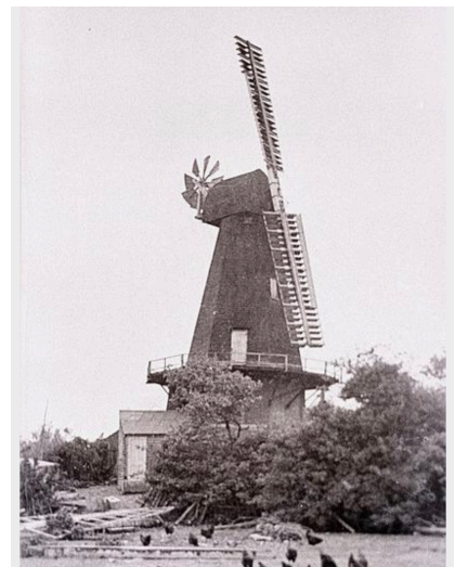
Figure 8: 1930. Two sweeps have been removed and the remaining pair have been slightly shortened.
