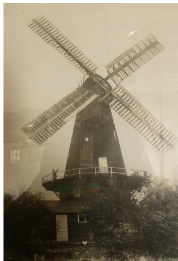
Figure 7: 1920s. The four patent sweeps have been widened so their leading and driving sides are equally wide.
