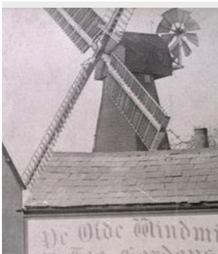
Figure 6: c1915. Two pairs of patent sweeps are now fitted. The 'leading side' of each sweep is narrower than the 'driving side', as is usual.
