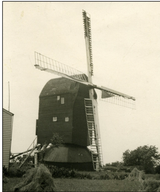
Figure 3: The post mill at Ash, Kent, fitted with the typical combination of a pair of common sweeps and a pair of shuttered sweeps.
