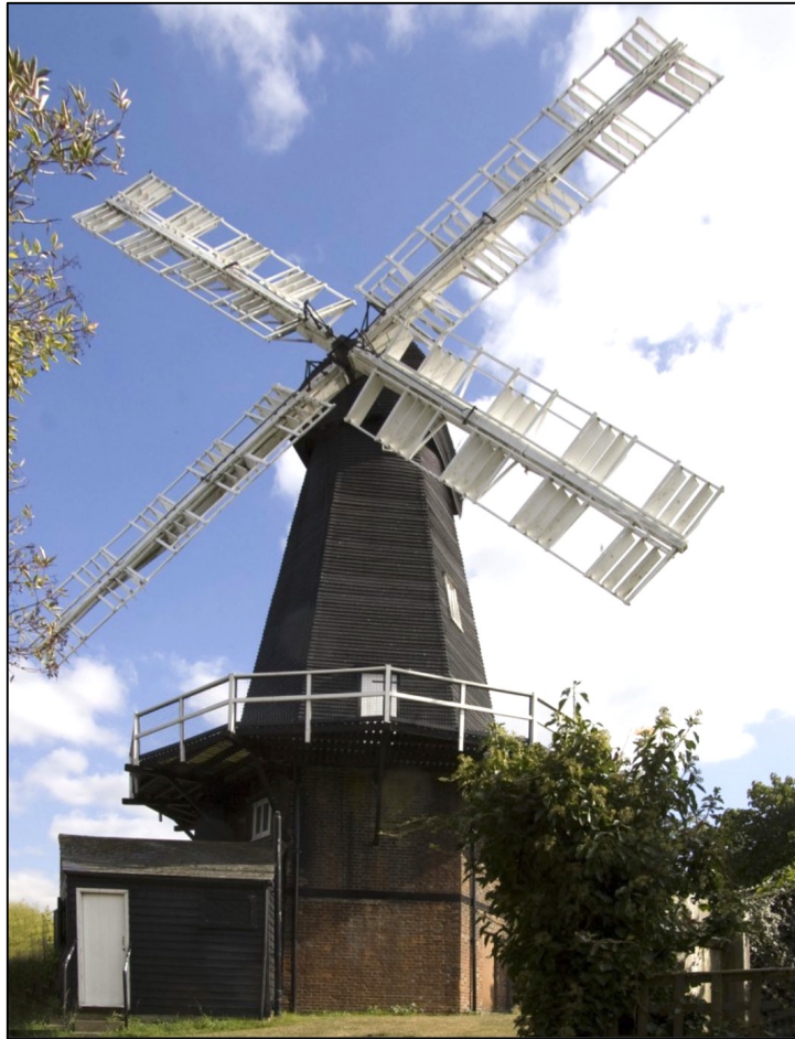
Figure 9: The mill in 2009, with oversized sweeps installed in 2003 (G Woodward).
