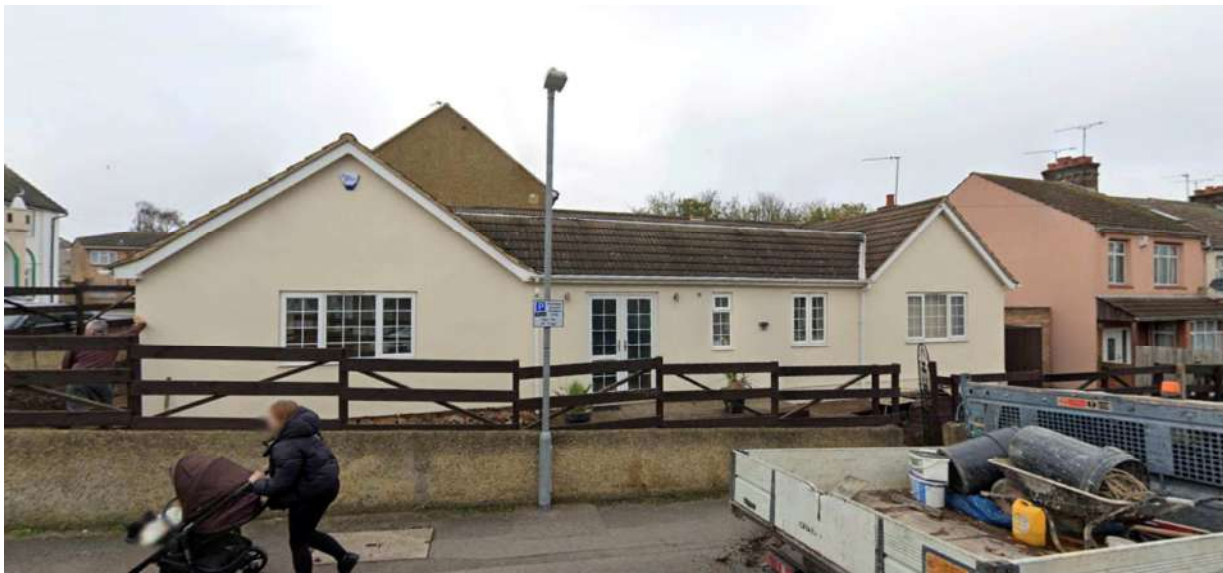
Existing bungalow viewed from Russell Road
