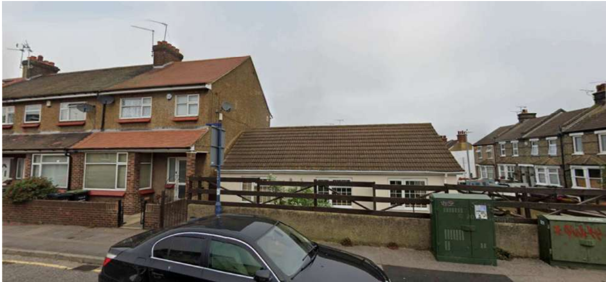
Existing bungalow viewed from Albion Terrace
