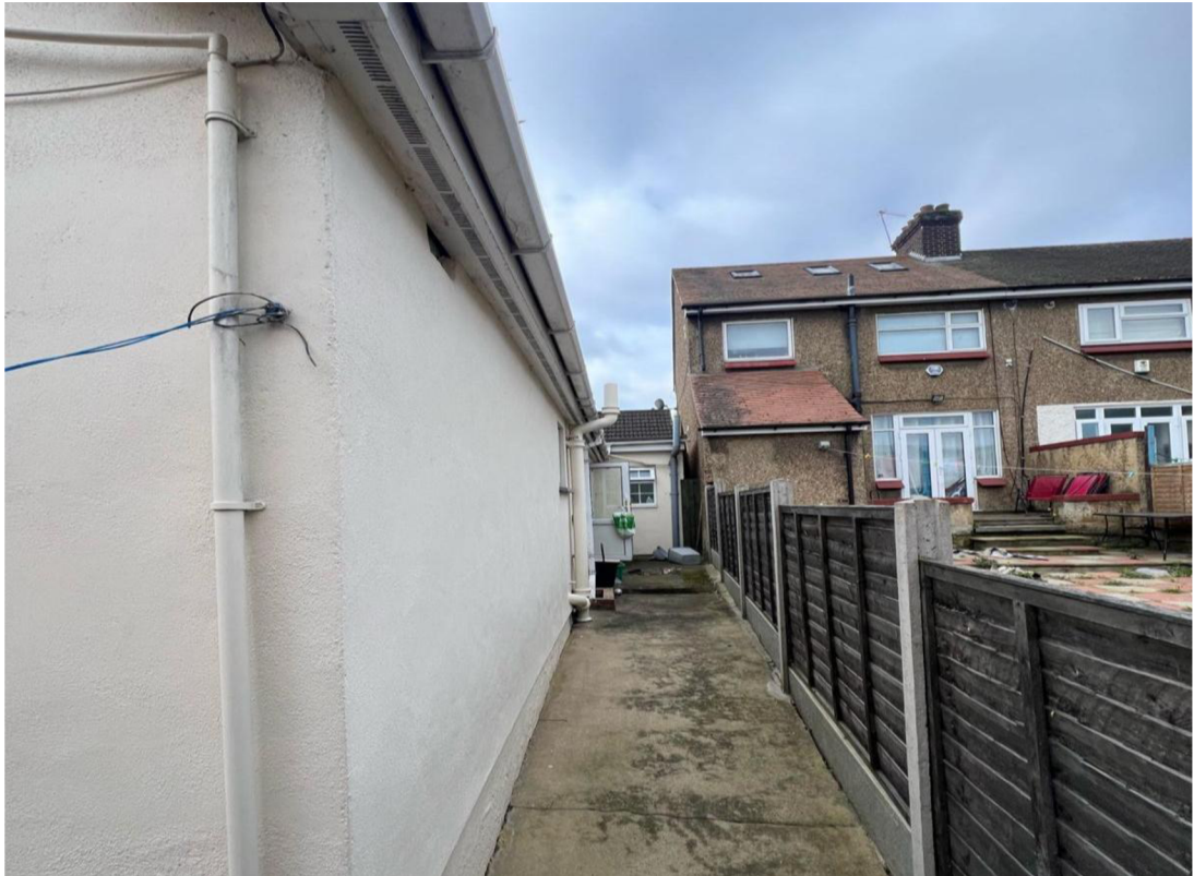
Image 7: Photograph of existing western boundary with rear elevation of No 25 Albion Terrace visible in background
