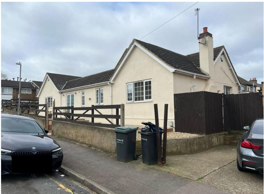
Image 6: Photograph of front elevation of existing property facing Russell Road.
