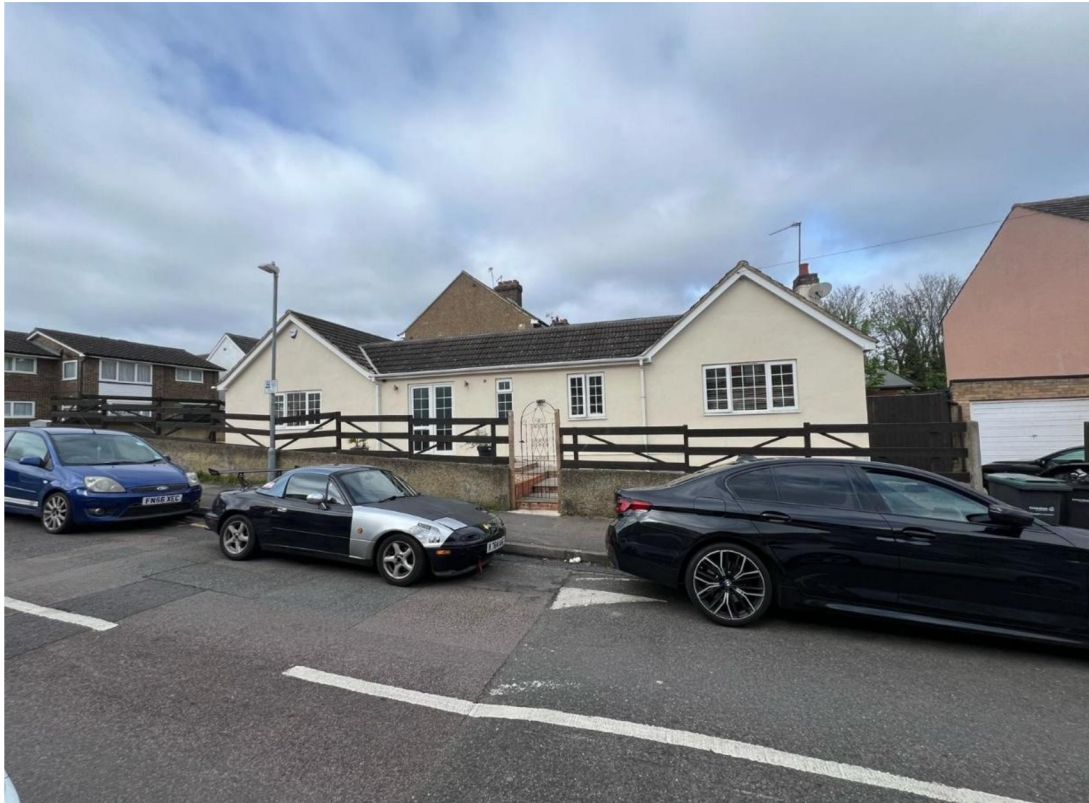
Image 3: Photograph of east elevation of site from Russell Road
