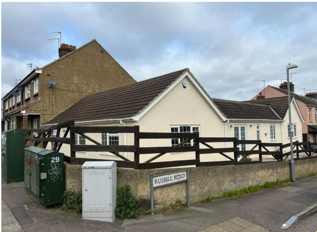
Image 4: Photograph of eastern and southern elevations of site as seen from corner of Russell Road and Albion Terrace. This image demonstrates how the existing property does not relate to the height/scale of the neighbouring terraces.
