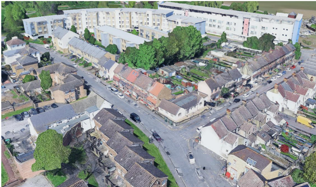
Image 2: Overhead view of site facing north west
