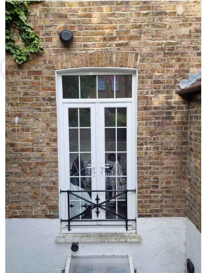
03. View of the current double doors, matching those at the front of the property in design, materials & proportion.
