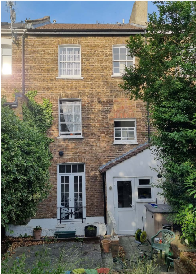
01. Stood at the back of the property in the private garden looking towards the rear facade.
