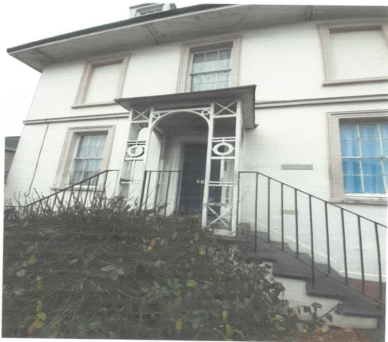
View of Porch From perry Street
