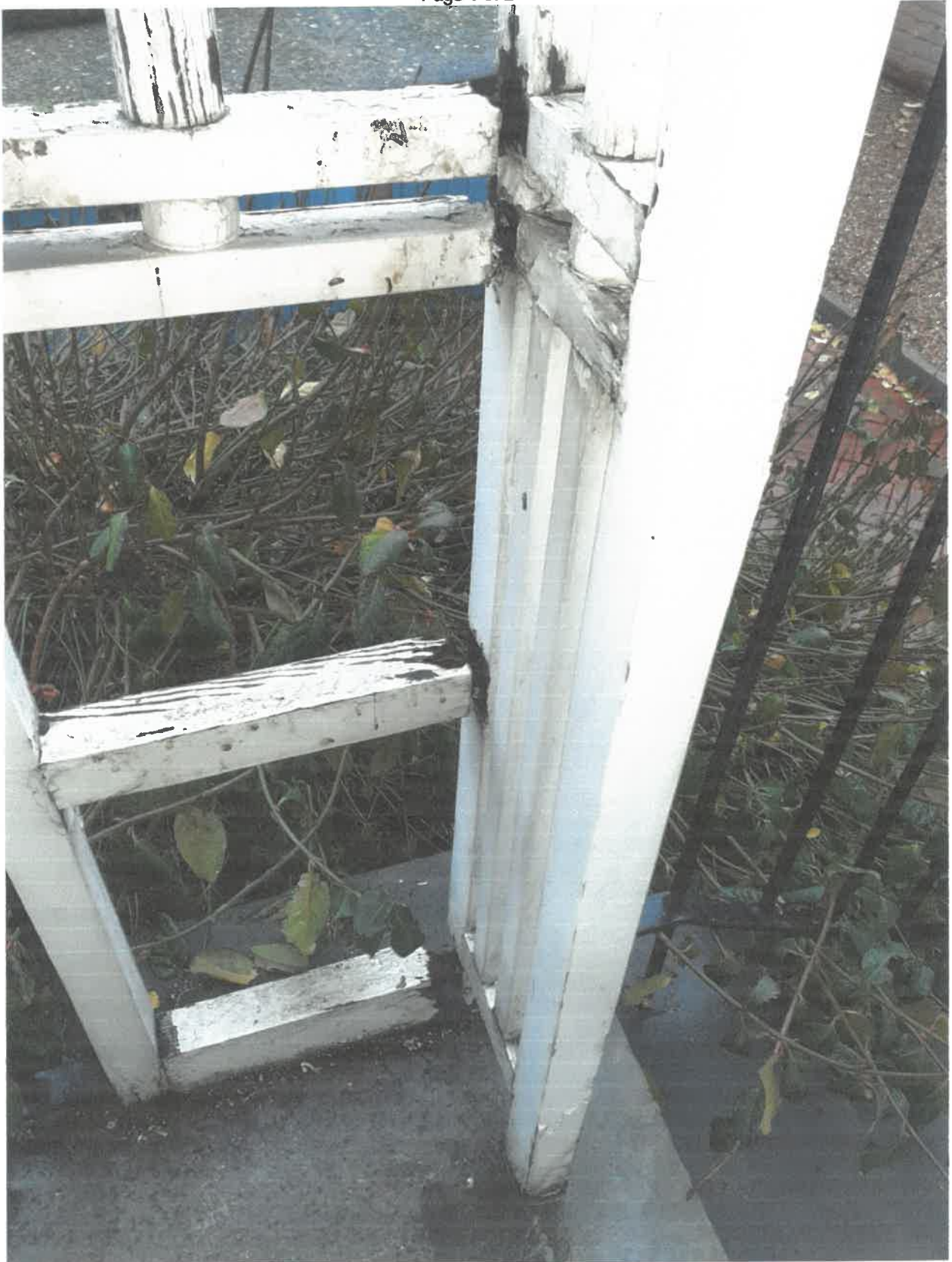
Typical condition of the timber frame that will be refurbished like for like
