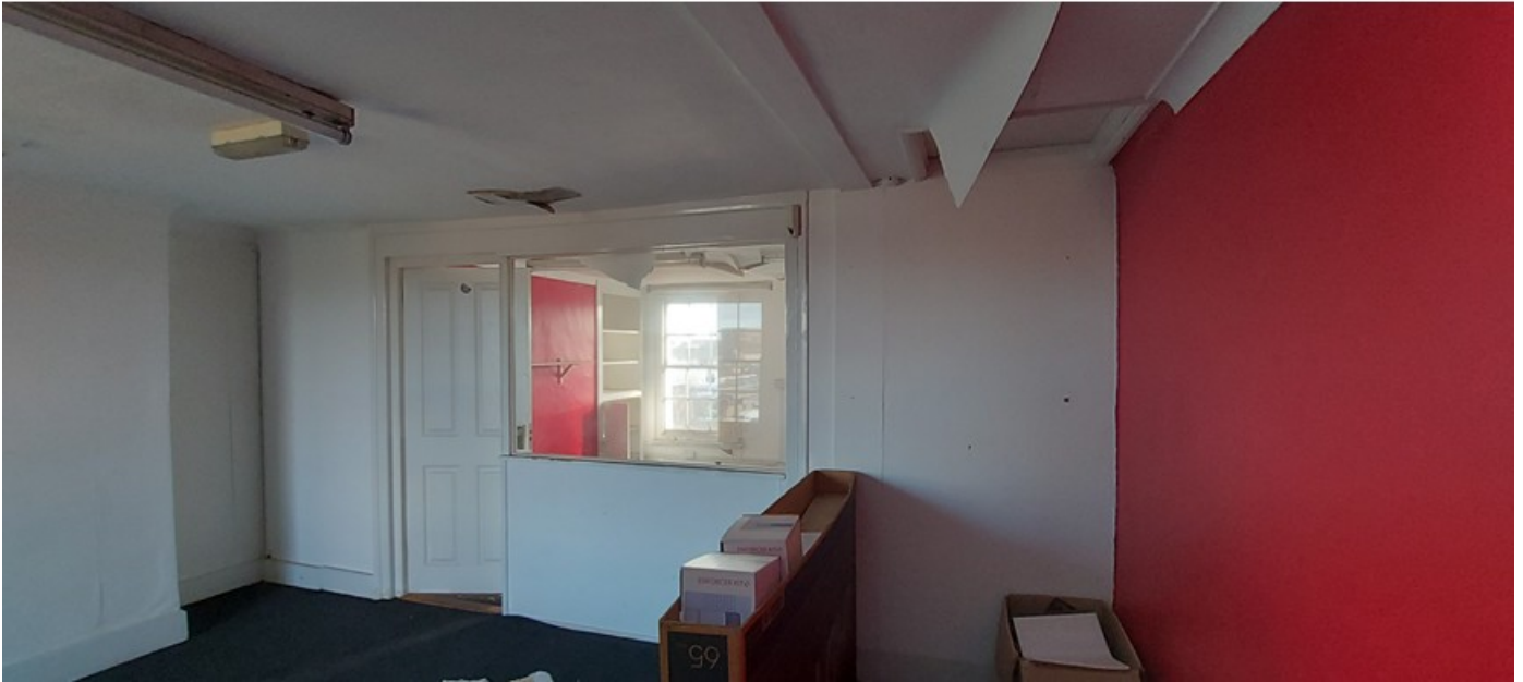
View from inside the rear room at second floor level looking towards the front room
