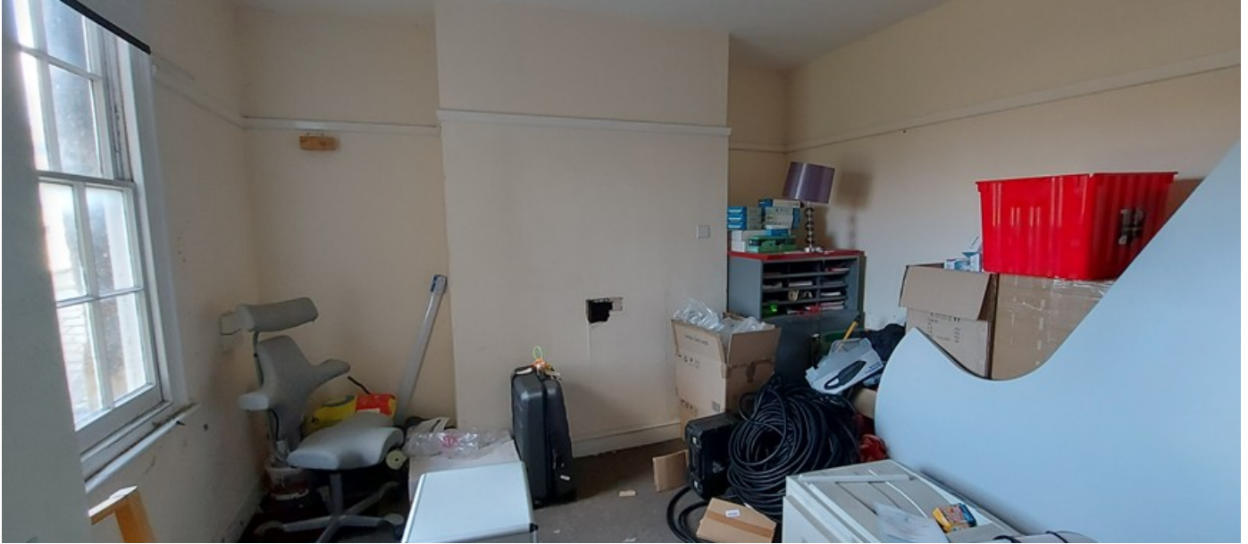
View from doorway of the first rear room looking inside, the dividing wall between the rear and front rooms is to the right
