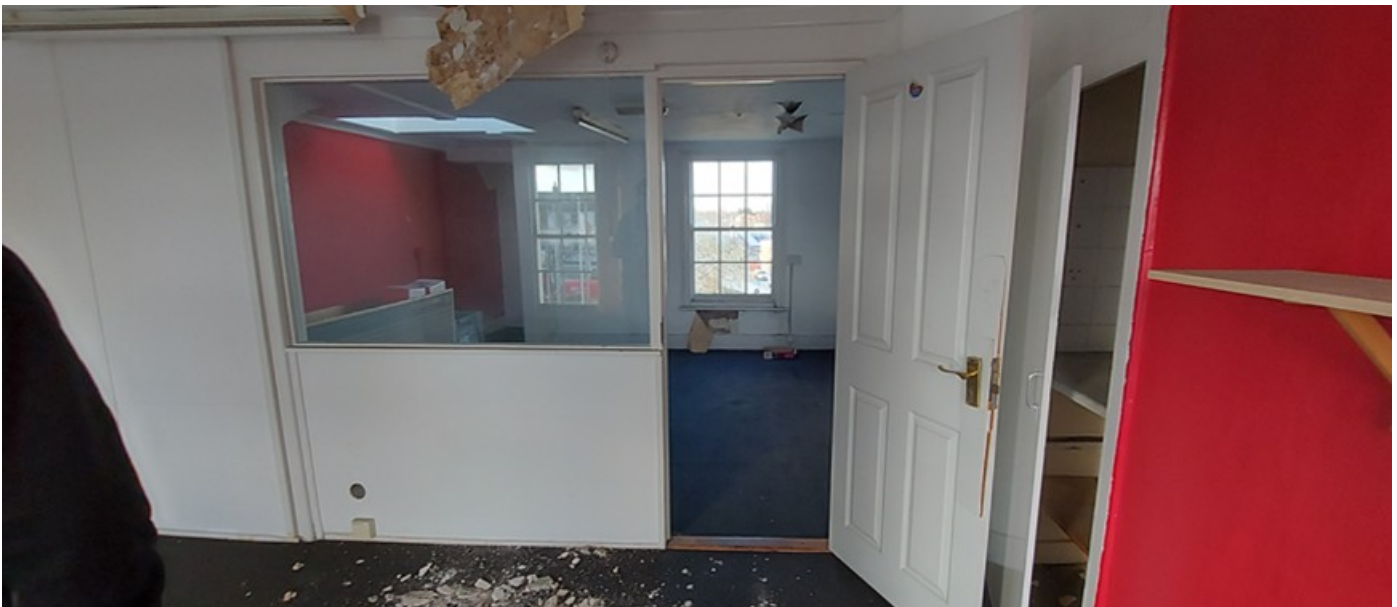
View from inside the front room at second floor level looking towards the rear room
